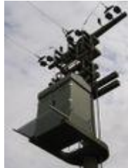
Masttrafostation
